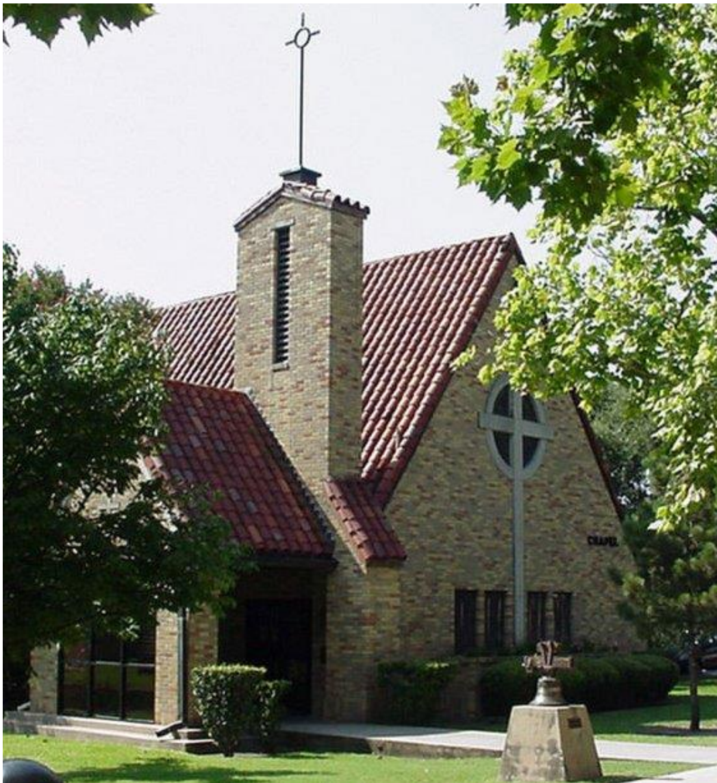
Serbin bell on concrete pedestal in front of Birkman Chapel, Concordia I-35
